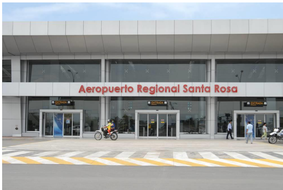
Figura 15 Aerpuerto Regional Santa Rosa
